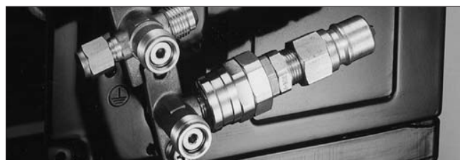
▲ Filling air conditioner refrigerant gas and pipe leak testing
