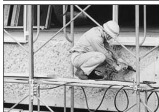
▲ Air pipe branching
